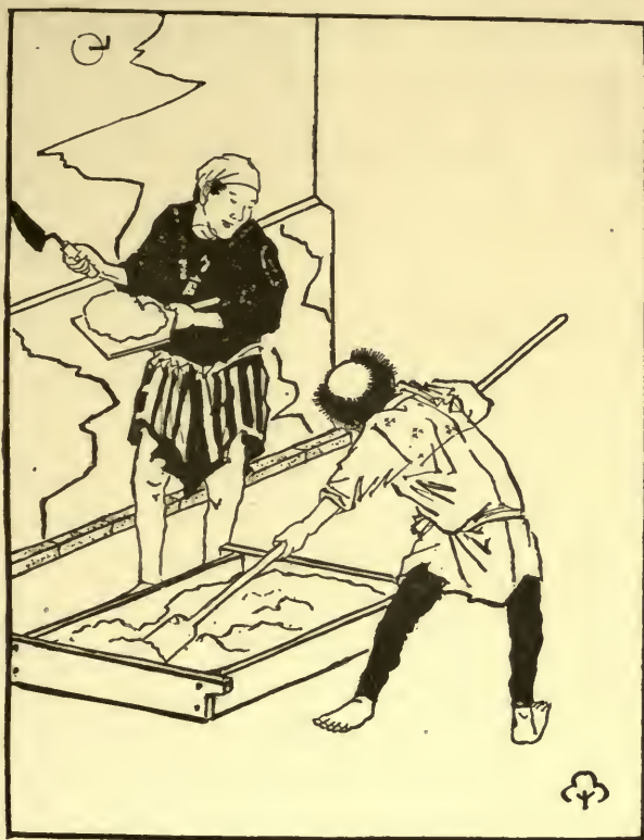
PLASTERERS AT WORK AFTER AN EARTHQUAKE.
